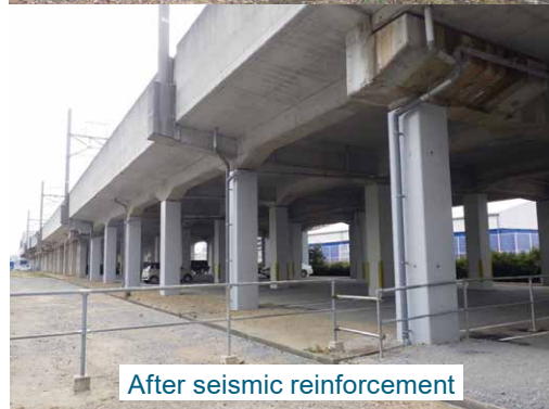
Example of seismic reinforcement for railway structures
