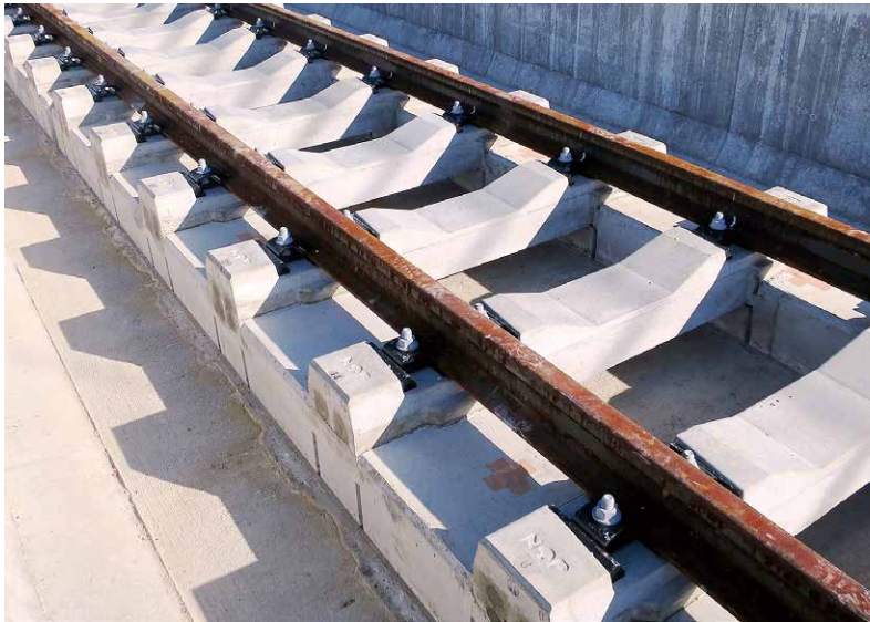
Solid-bed track equipped with resilient sleepers using the shear-key
