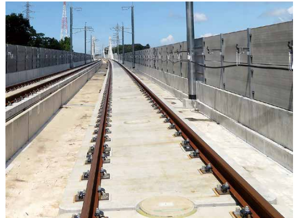
(b) Example of a slab track being laid
