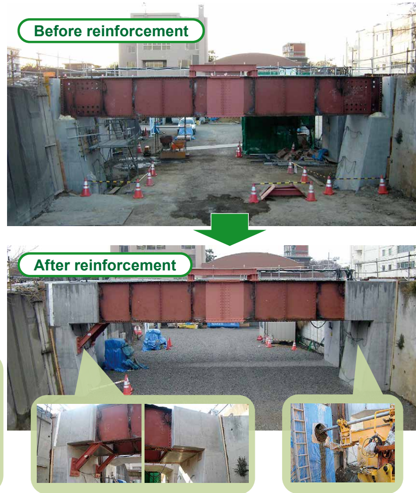
Seismic reinforcement technology of steel railway bridges (Integration of bridge girder, abutment, and embankment)
