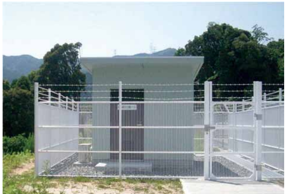
Detection points are located along railway tracks or quiet places distant from tracks. Constant temperature and humidity are maintained inside the buildings housing seismometers in order to ensure stable operation of the seismometers over a long period.
