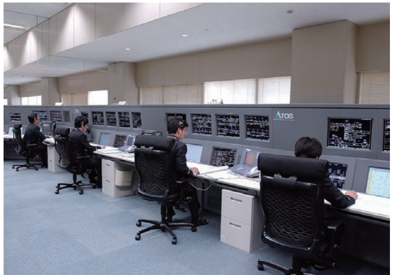
Autonomous Decentralized Transport Operation Control System of JR East (courtesy of JR East)
