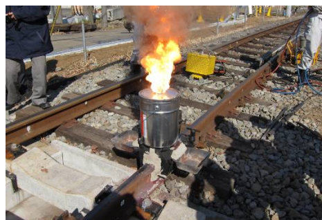
(a) 溶接施工
