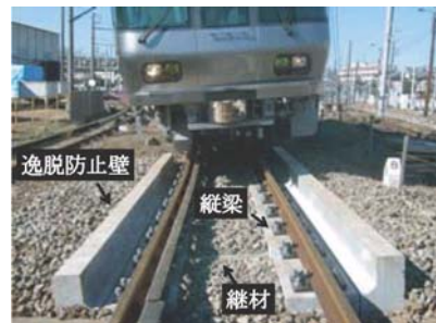
(c)敷設状況
