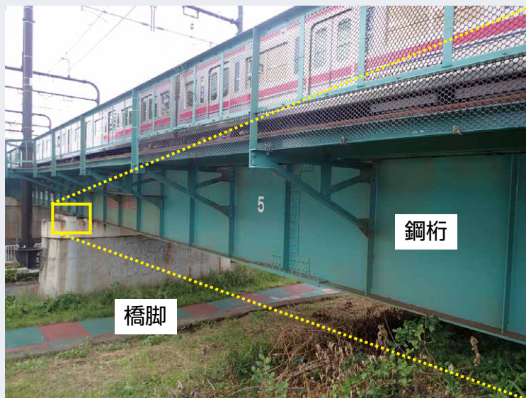
図1 鋼桁の支承
