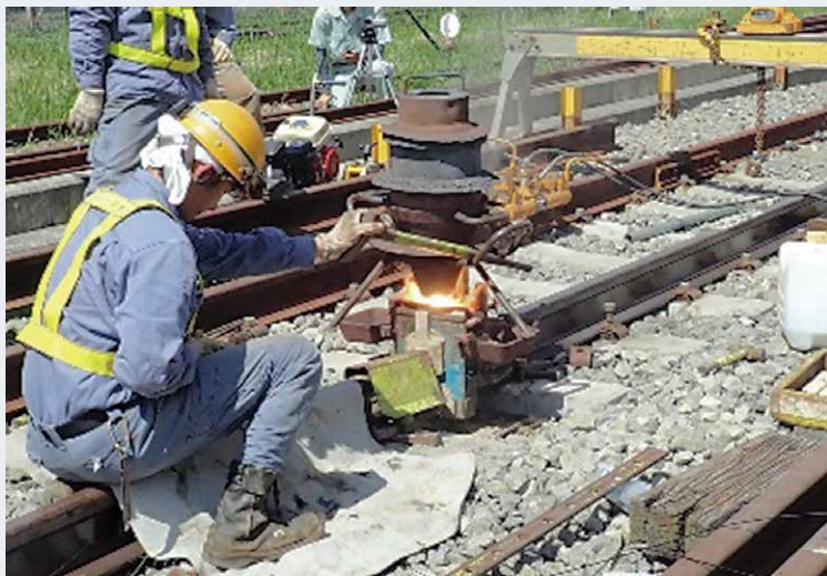
(a) 溶接状況
