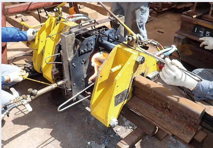
(a) 溶接状況
