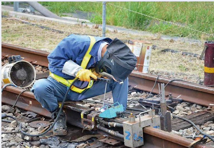
(a) 溶接状況
